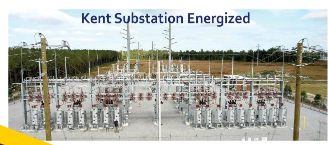
Powered Up! OREMC's new 230 kV Kent Substation-a joint venture with FPL at the Crawford Diamond Industrial Park in Callahan-is energized. Two of the six circuits are serving West Nassau County, providing room to grow and increased capacity, as well as system redundancy to facilitate enhanced reliability.
